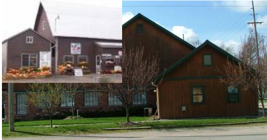
Genson's Plumbing Store (Potential Cider Mill or Restaurant)
