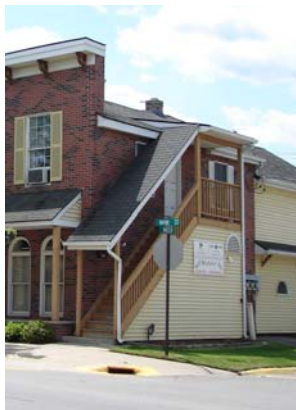
Avoid open air exterior stairwells
